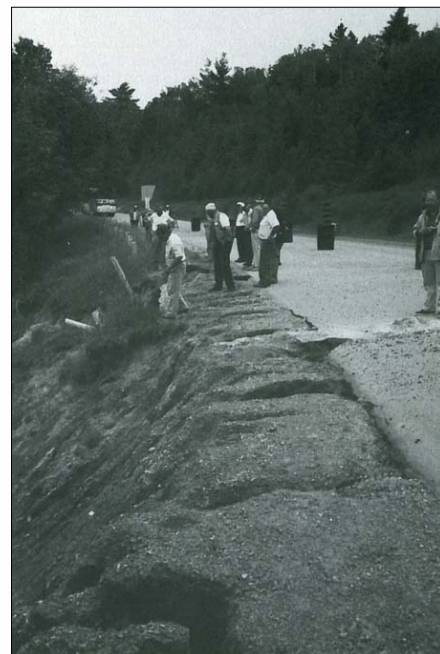
Before (above), after (below): In the 1980s, the NVCA and the County of Dufferin repaired the riverbank along a stretch of Hockley Road that had been eroded by the river.
