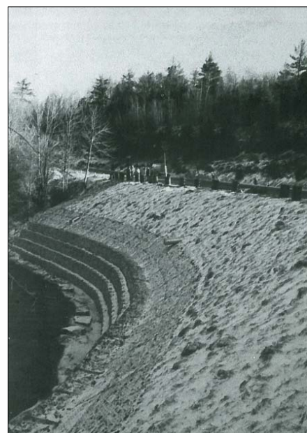
Before (above), after (below): In the 1980s, the NVCA and the County of Dufferin repaired the riverbank along a stretch of Hockley Road that had been eroded by the river.
