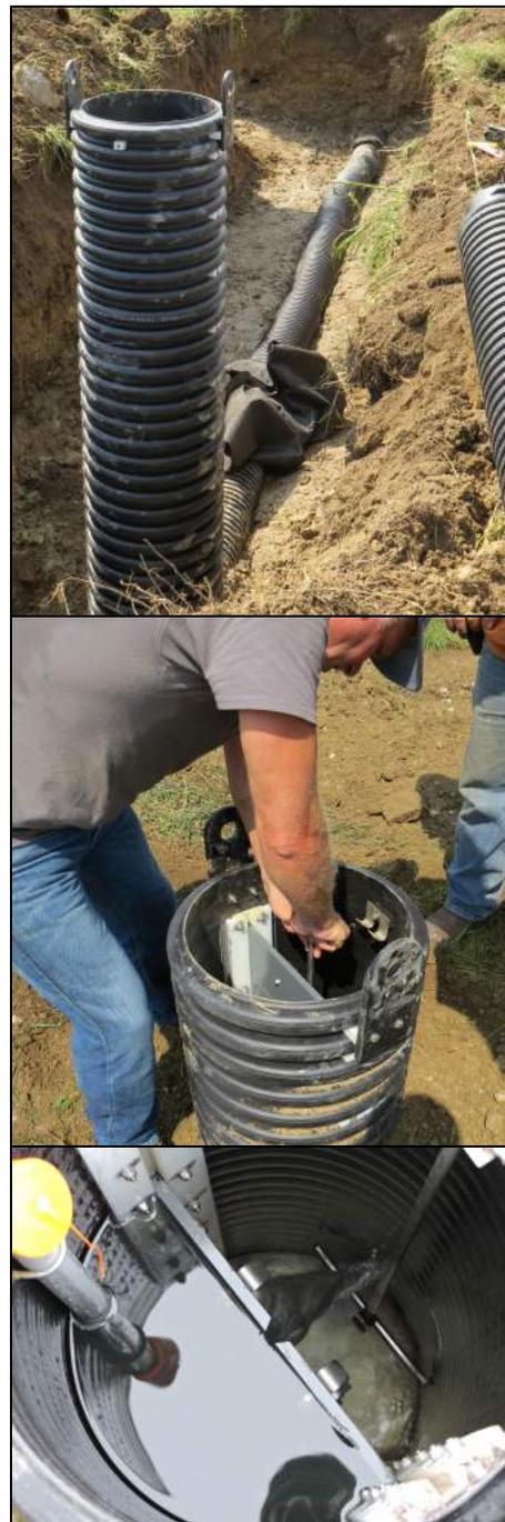
Top: Installation of a control structure. Middle: Adding stop logs to raise the water table. Bottom: The interior of the control structure, showing the raised water table controlling drainage. Photos: UTRCA.
