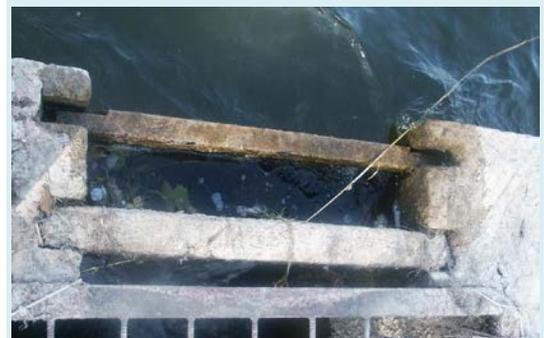
*If your ponds drop-well already contains two-slots for stop-logs, it can be easily modified to become a bottom-drawing pond. Hemlock is the wood of choice for stop-logs.*
