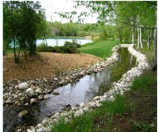
*This new bypass channel separates the pond from the stream. This improves water quality downstream, and lets fish migrate to spawning grounds. It also slows the sedimentation of the pond, which extends the life of the pond.*
