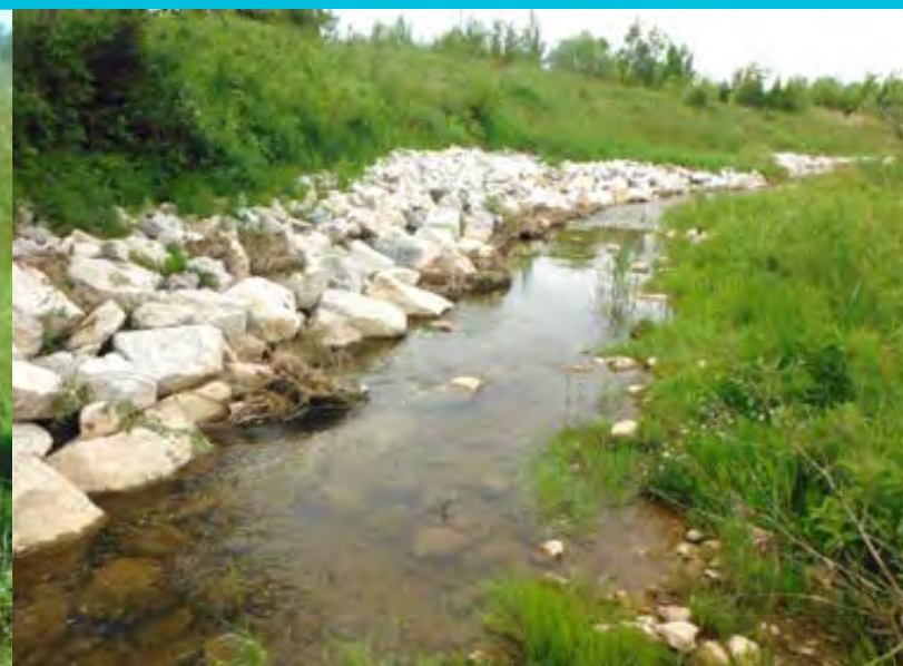
An example of streambank restoration in the Blue Mountains subwatershed: Trout stream restoration and bank stabilization in constructed floodway, Black Ash Creek Collingwood.
