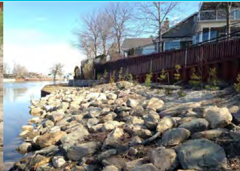
An example of streambank restoration in the Lower Nottawasaga River subwatershed: Construction of a habitat friendly shorewall project on the lower Nottawasaga River, Town of Wasaga Beach.
