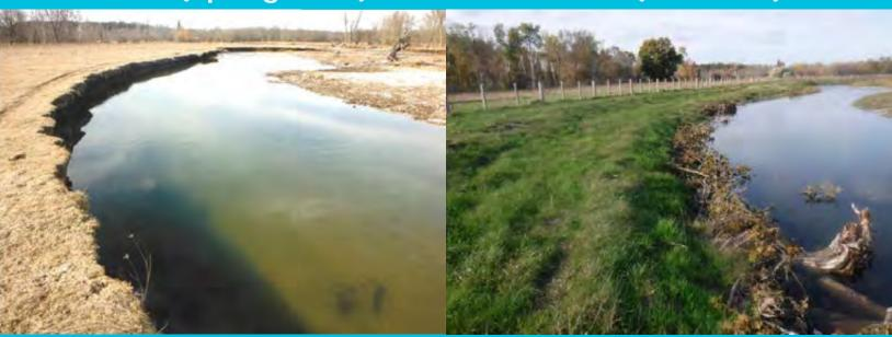
An example of streambank restoration in the Upper Nottawasaga Valley subwatershed: Example of a restoration project on the Upper Nottawasaga River which included installation of livestock exclusion fencing and habitat friendly streambank stabilization.
