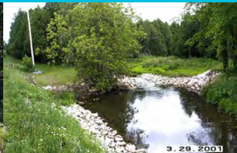
An example of streambank restoration in the Boyne River subwatershed: Example of historic dam removal project on the Boyne River designed to provide for fish passage and improve water quality.
