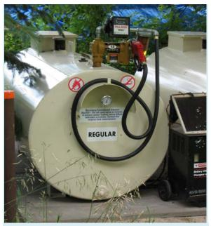
A ULC approved double-lined tank with a vacuum gauge, protected from vehicles by safety-bollards helps prevent spills and safe-guards our drinking water.
