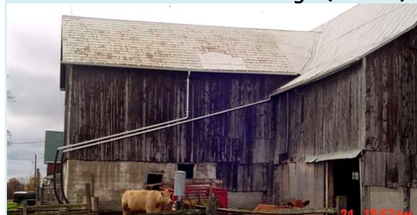
Steel eaves funnel clean rainwater into a big-O pipe that directs water into a swale away from the barn and livestock yard.
