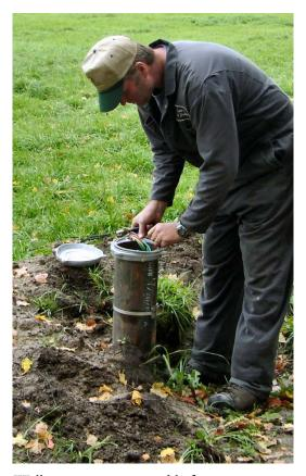
Well owners are responsible for maintaining their wells to prevent the entry of surface water or other material. Annual maintenance and visual examinations should identify and fix problems such as sunken earth around the well and missing well caps.
