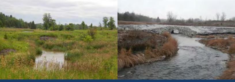
An example of stream restoration in the Innisfil subwatershed: A retrofitted failed ice dam structure completed to reestablish a fish migratory route and maintain cool water in Beeton Creek.
