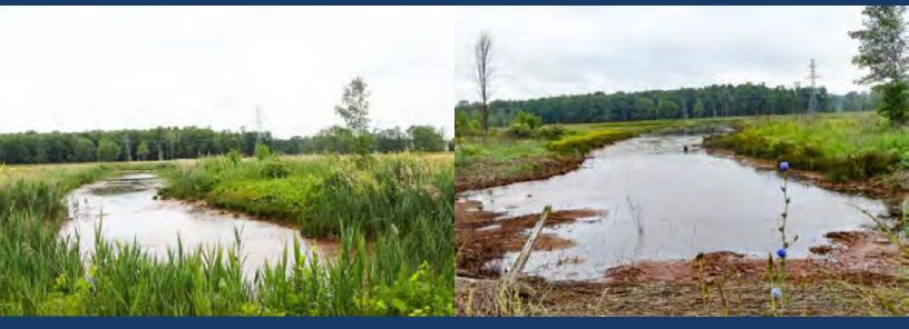
An example of streambank restoration in the Mad River subwatershed: Trout stream restoration and bank stabilization in constructed floodway, Black Ash Creek Collingwood.
