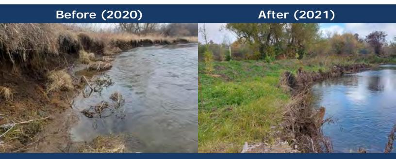
An example of streambank restoration in the Upper Nottawasaga subwatershed: The slumping banks of the Upper Nottawasaga River was restored to decrease erosion, improve water quality and provide fish habitat.
