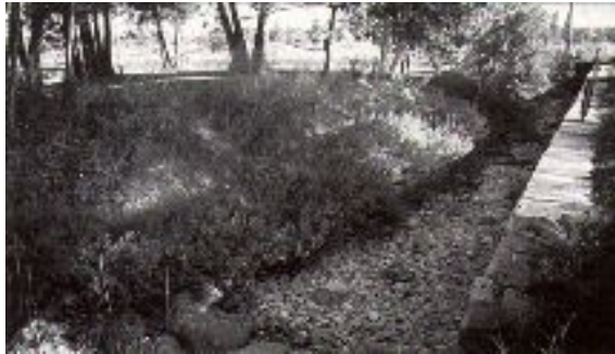
Photo 5 - Summer 1995 The crib wall is approaching the second year of growth. The willows are growing vigorously, thus providing protection and stability for the stream bank
