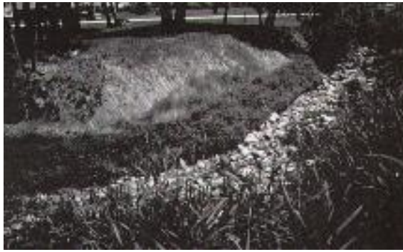
Photo 4 - Spring 1994 The crib wall is starting to grow. Note how the willows are developing
