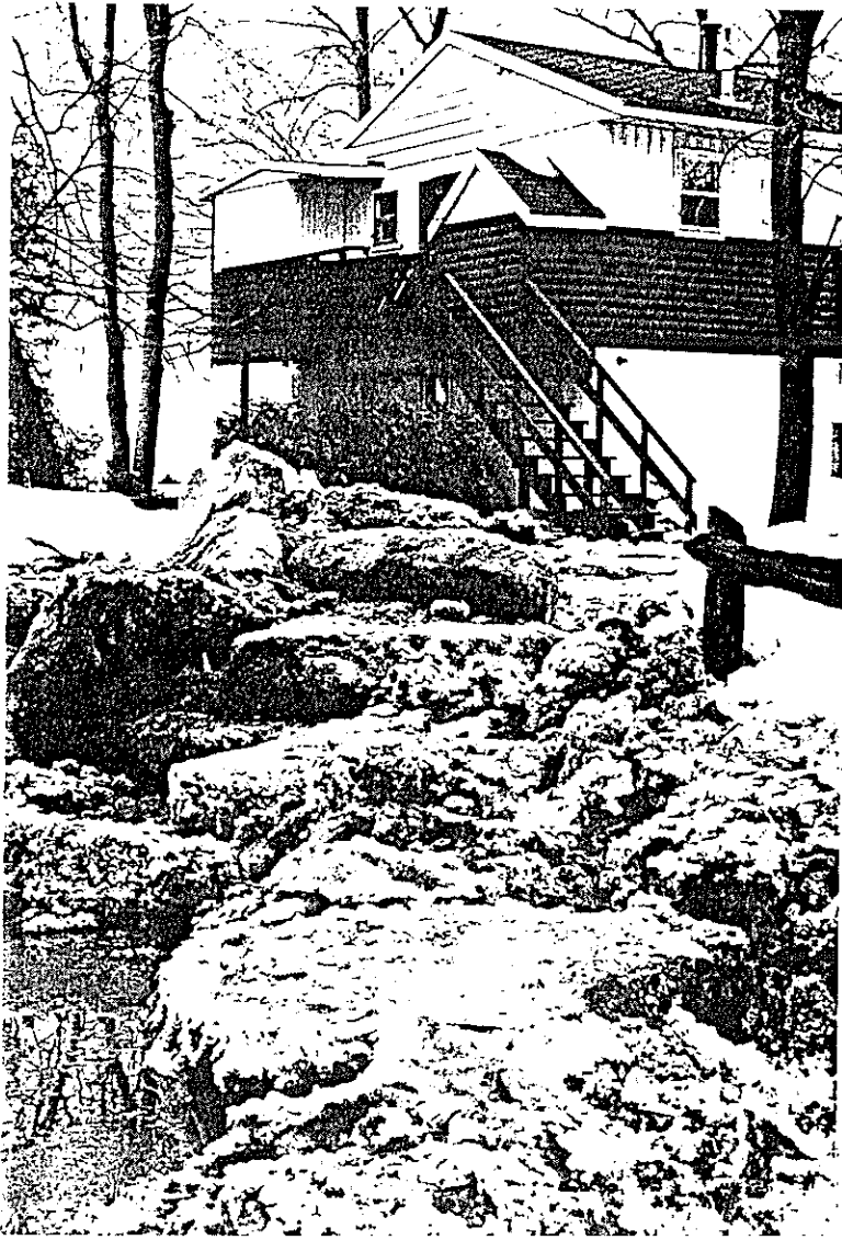
Grounded Chunk Ice Encompassing Residential Dwelling
